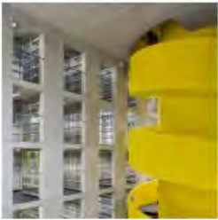
Baukuh's House of Memory features a decorative facade and a monumental yellow staircase
